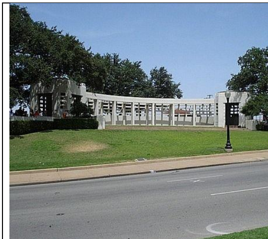
The concrete pergola on the grassy knoll
